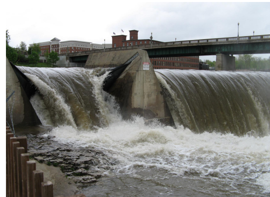
Winooski, VT - Winooski One Hydro Electric Facility
