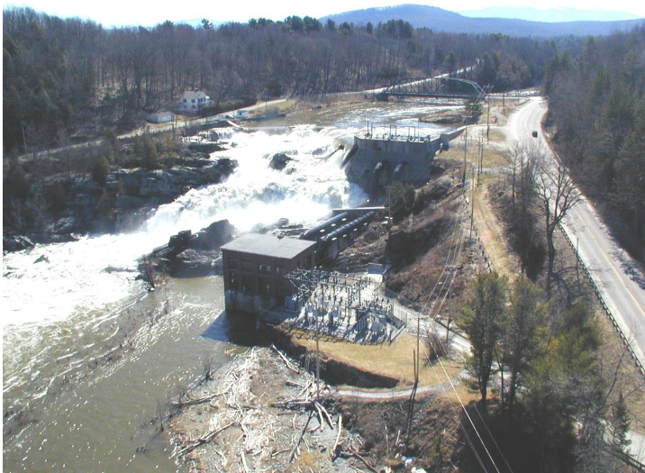
Fairfax, VT – Hydro Facility Owned & Operated by CVPS
